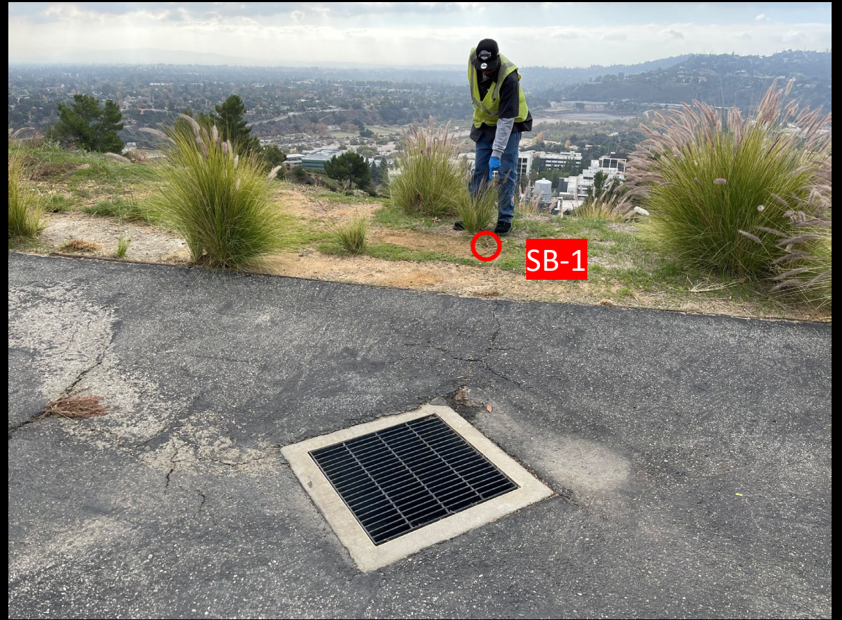
Storm Drain and Sample Technician Pointing at SB-1 Location
